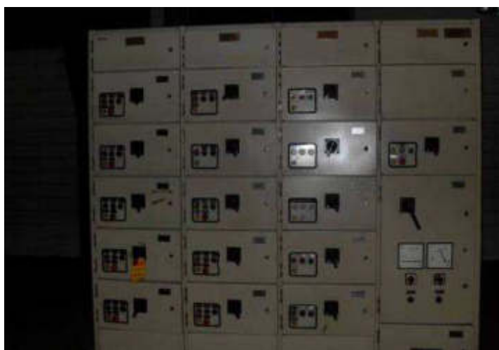
Figura 166 - Painel do CCM – 460 V
